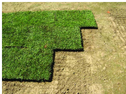
Figure 4. On each row of sod, stagger the joints as when laying bricks.
