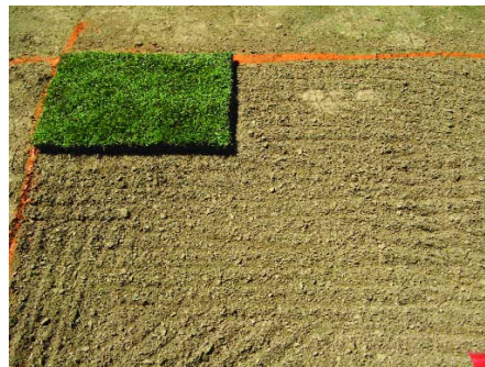
Figure 3. Install the first piece along a straight edge.
