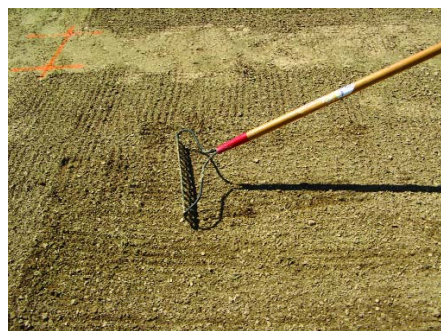
Figure 2. Loosening the soil to a depth of 0.5 inches prior to sod installation helps with rooting.
