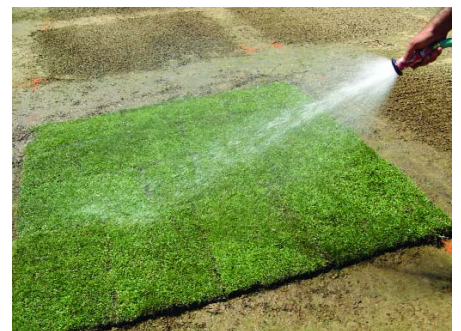
Figure 6. Begin to water the lawn thoroughly after the sod is installed and rolled.
