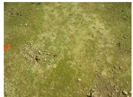
Figure 1. Bare soil clean of weeds prior to sod installation.
