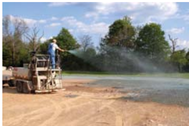
Figure 5. Arkansas lawn being established by hydroseeding.
